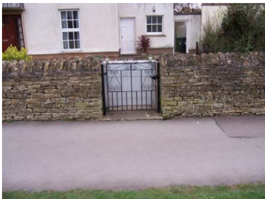
Flood defence as seen from the road gateway cover deployed as necessary.
