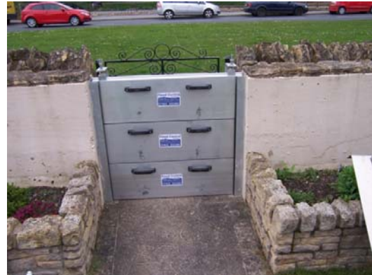
Flood defence as seen from the front of the house - gate blocked off during a flood
