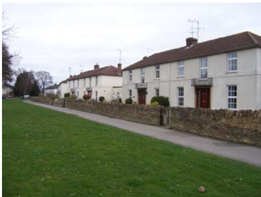
View of flood wall along the frontage of the properties
